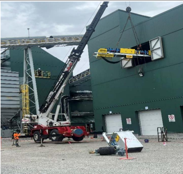
Figure 3: Installation of the third ore sorter conveyor, external view
