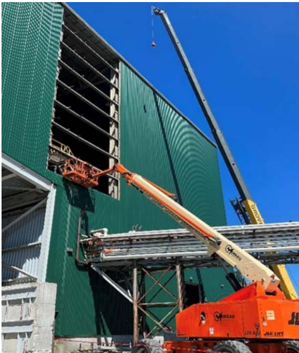
Figure 1: Opening for the WHIMS installation
